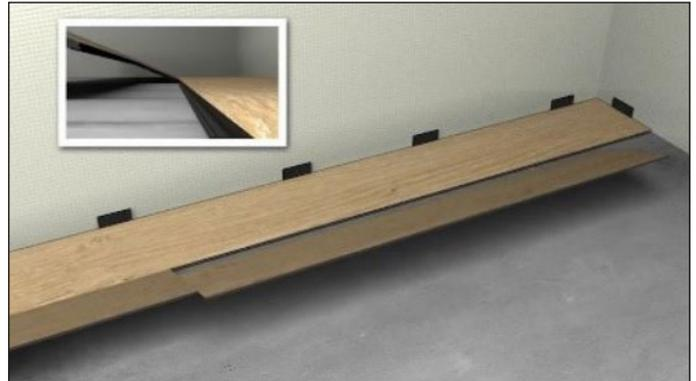
5. Gently slide the new plank down so that the tongue of the new board is engaged tightly into the indent of the existing plank in the previous row.
